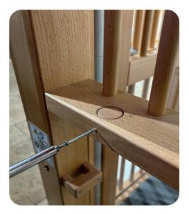
7 Screw the plug in place with the enclosed screws without pre-drilling.
